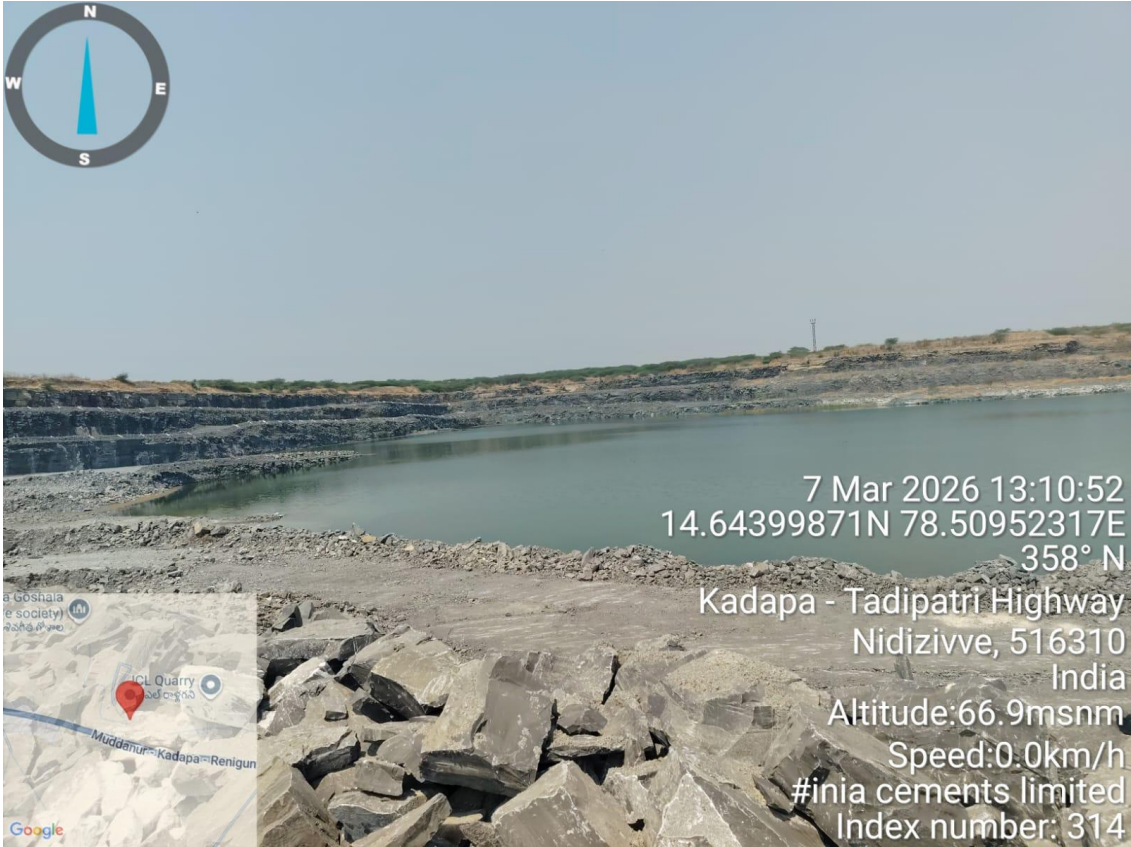
Block-1 in Limestone mine of M/s. The India Cements Ltd.
